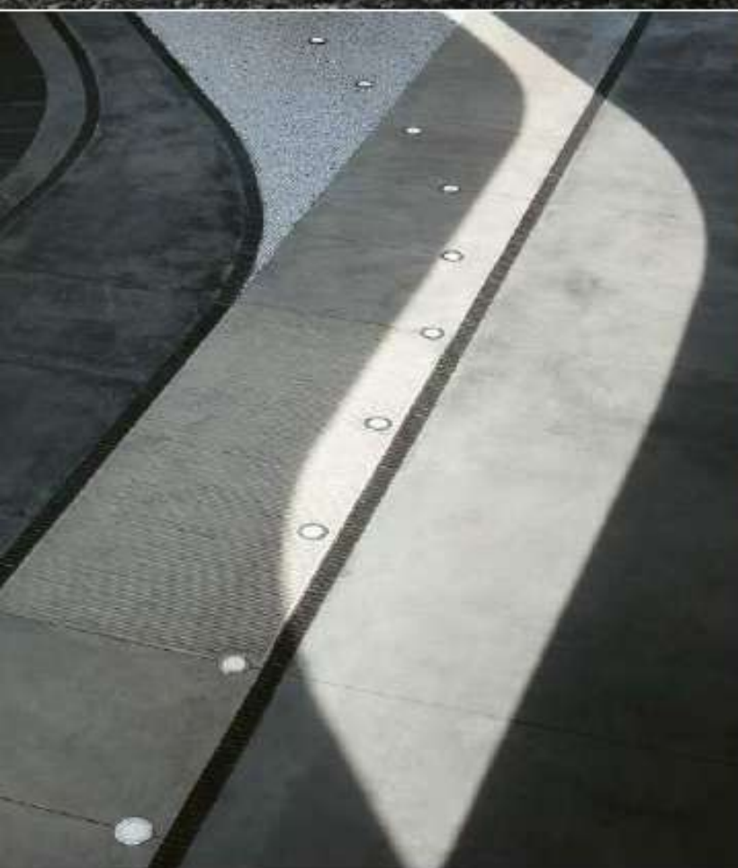
Location luminaires and floodlights specially for flush-mounting installation in paved ground surfaces
